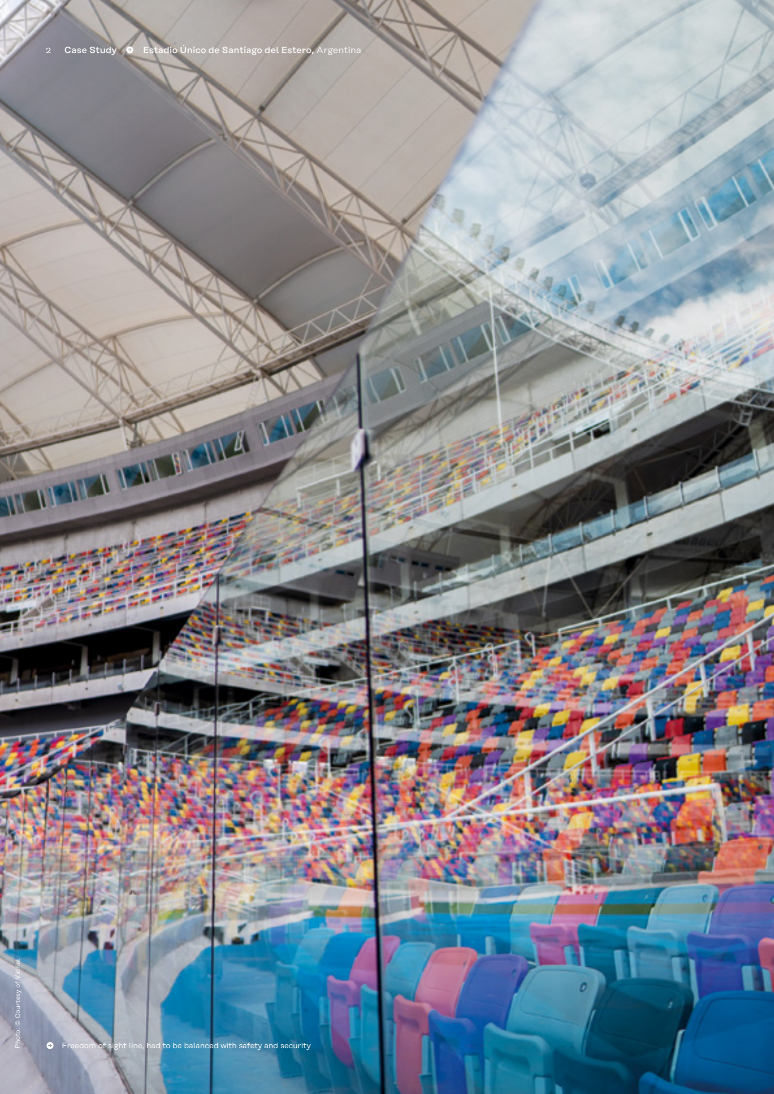
The balustrade panels are fabricated from 10 mm fully tempered glass + SentryGlas® + 10 mm fully tempered glass
